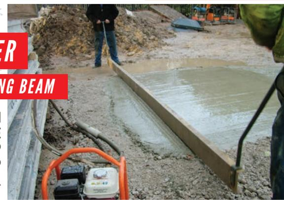
A MANUALLY-OPERATED LIGHTWEIGHT ALUMINIUM TAMPING BEAM DESIGNED FOR COST-EFFECTIVE LEVELLING OF CONCRETE PADS. THE HAND TAMP REQUIRES TWO OPERATIVES TO MANUALLY TAMP AND DRAG THE CONCRETE TO THE FINISHED LEVEL.
